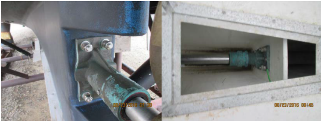
Photo's 11 & 12 (Stuffing Box and Shafting)
